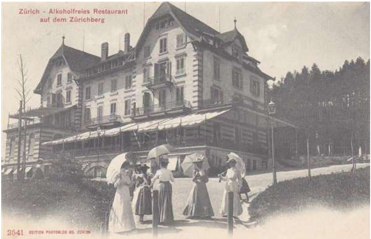
Rest. Zürichberg, Orellistr. 21, 8044 Zürich (1908)
